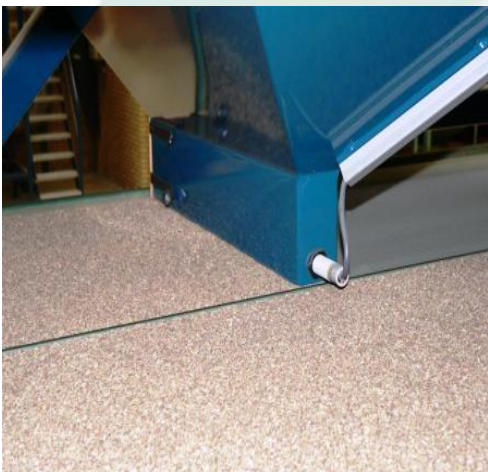
Seed supply belt hopper bin installation.
